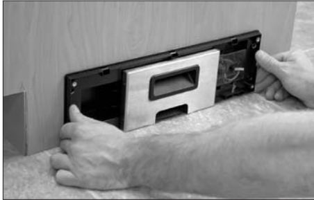
11 Unit in place.
