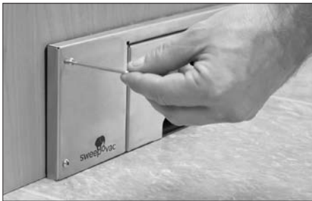
13 Screw on the face plate.
