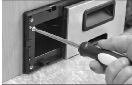
12 Screw into place using the 4 wood screws.
